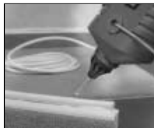
Laying telephone cable.
